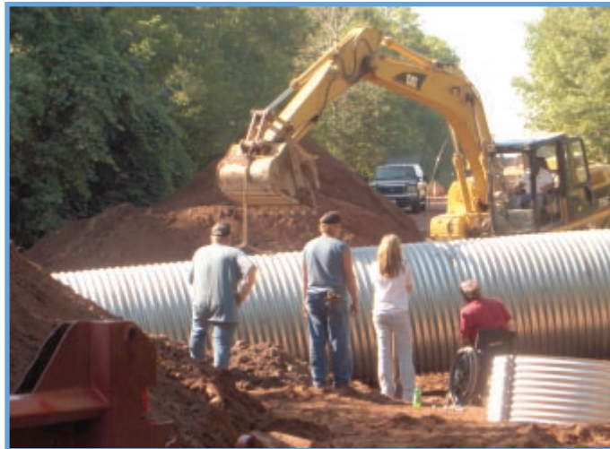
The Bad River Watershed Association assists towns in finding funding for culvert replacement to protect water quality. Here, a new culvert is installed in the Town of Ashland.
