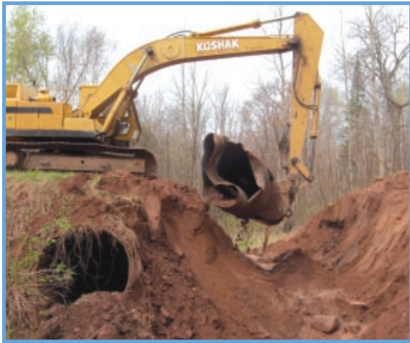
The Bad River Watershed Association assists towns in finding funding for culvert replacement to protect water quality. Here, a new culvert is installed in the Town of Ashland.
