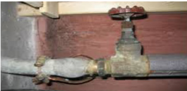
Picture of lead service line entering a household
