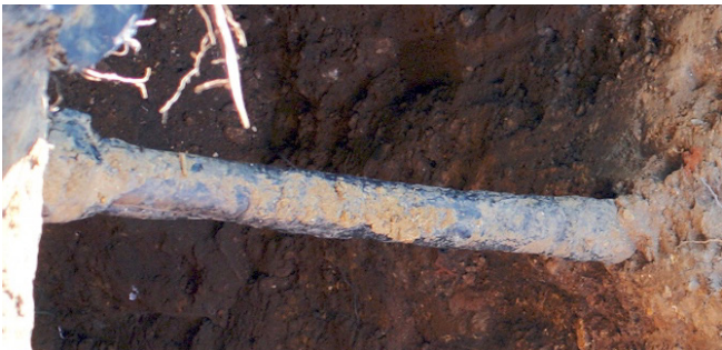
Picture of a lead service line
