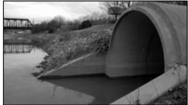
Any moderate to heavy rain storms lead to the dumping of untreated sewage into our waterways from pipes like this one on Ohio's Scioto River.
