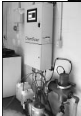
Sanitary sewer overflow meter and location of the overflow tank at Bellevue Park, Sault Ste. Marie. Photos by Carol Martin.
